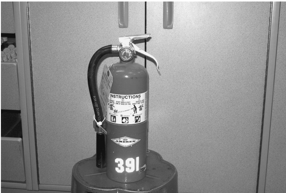
Figure 10-10 Portable extinguishers are marked to indicate what type of fire they should be used on.
