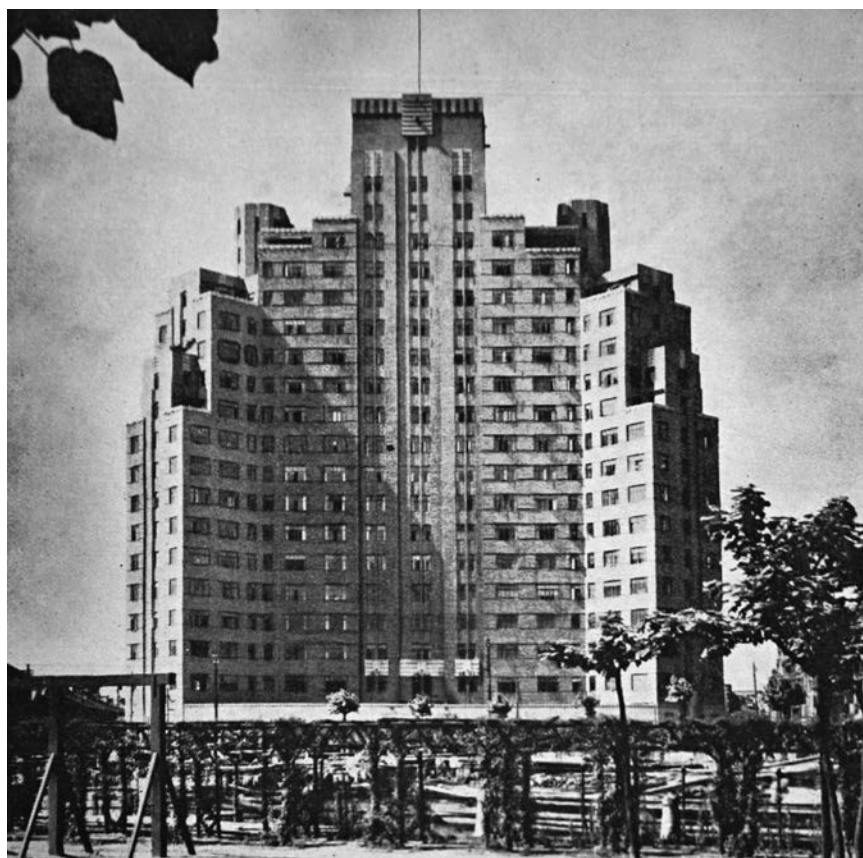
Figure 9.5 Broadway Mansions (1934), Shanghai, designed by Bright Fraser and Palmer & Turner.
