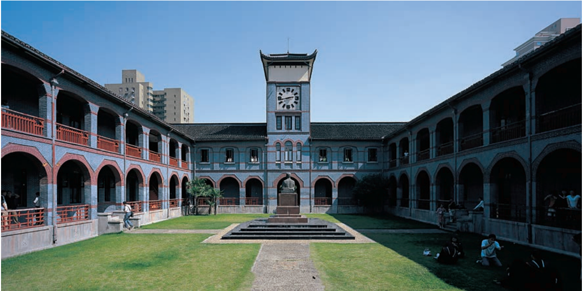
Plate 16 St John's University, Shanghai, designed by Atkinson & Dallas.
