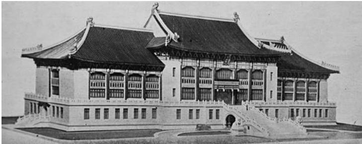
Figure 1.8 Model of the Mayor's Office (1934), one of the principal modern buildings in Shanghai's Civic Centre, designed by Dong Dayou.
