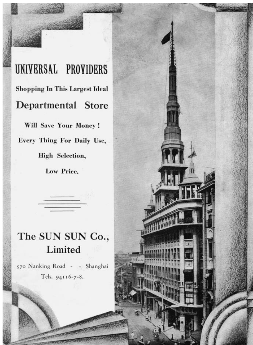
Figure 9.15 Sun Sun department store (1926), designed by Charles Gonda.
