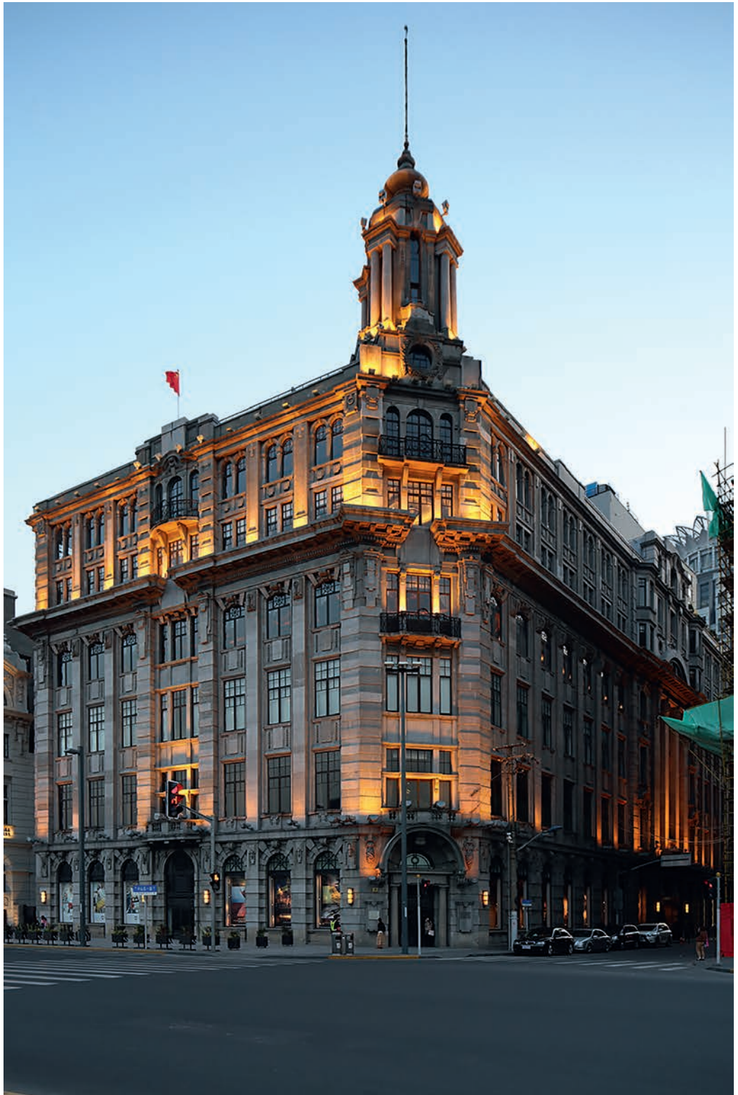
Plate 13 The Union Assurance Company of Canton (1916), designed by Palmer & Turner.
