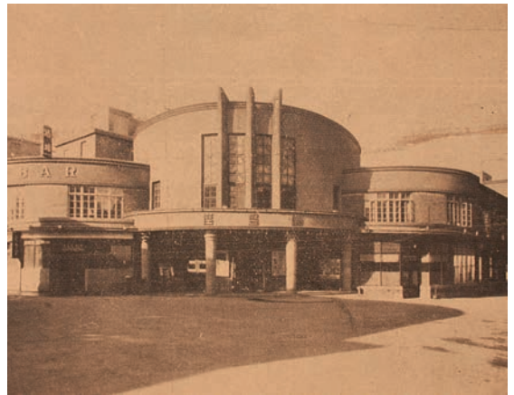
Plate 10 The Tokiwa Cinema (1932), Dalian, designed by Munakata Architectural Office.
