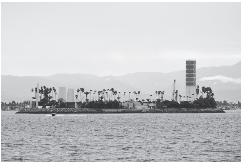
FIGURE 11. A Long Beach oil island, with the shoreline in the far background, 2018. Built in the 1960s, the four oil islands were designed with visual aesthetics that would disguise industrial activity, but they are massive oil drilling platforms. Photo by Ian E. Abbott, CC-BY-NC-SA 2.0 license.
