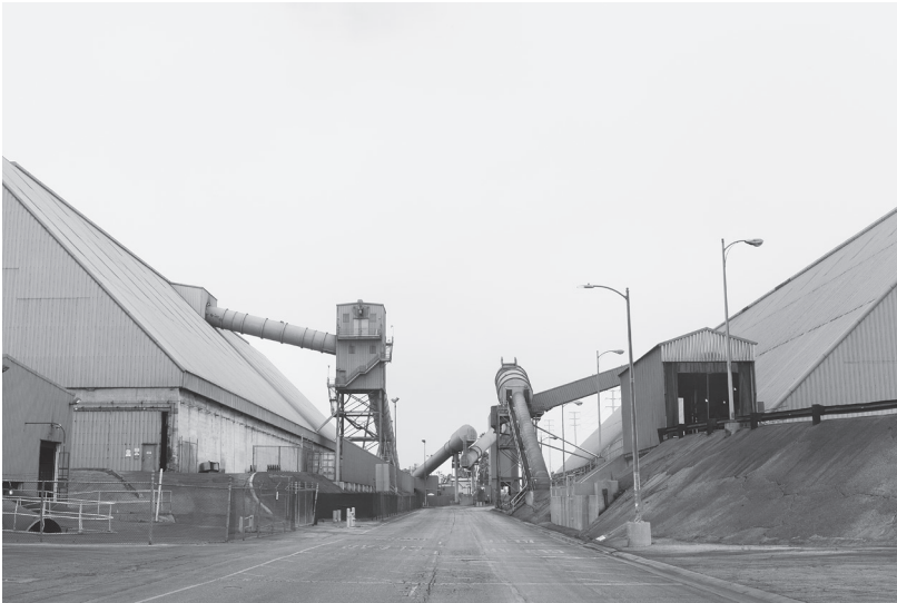
FIGURE 29. Petcoke handling facilities, which today must be covered so toxic dust will not blow onto residents. Port of Long Beach, 2021. Photo by McKenzie Stribich.
